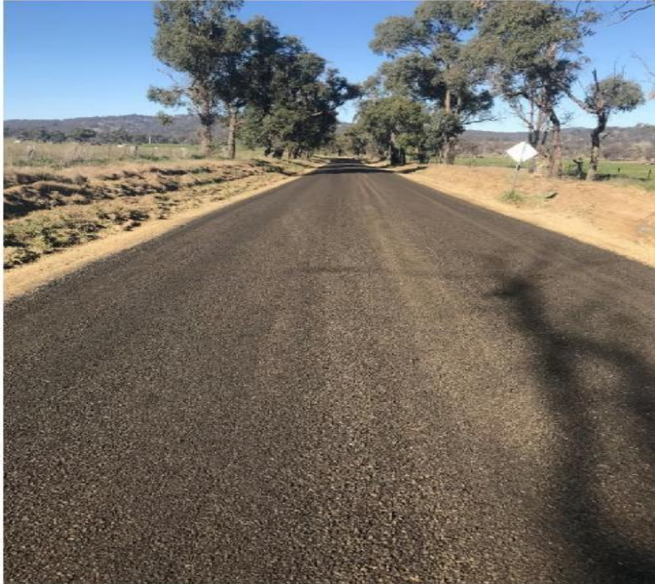
Image: Graded Aggregate Seal on Yarraford Road
