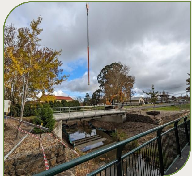
Image: Construction of Wentworth Street bridge
