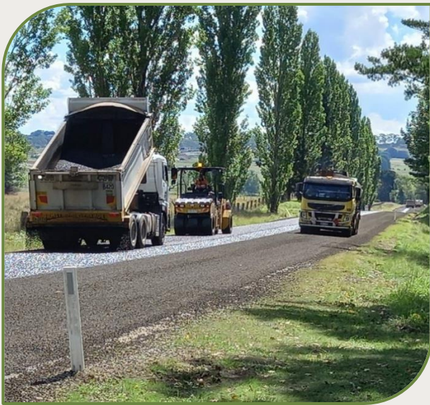
Image: Rehabilitation Works Shannon Vale Road
